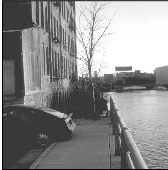
141 North Water St. - New Condominiums
