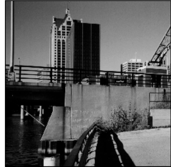
Grade Change at Bridge
