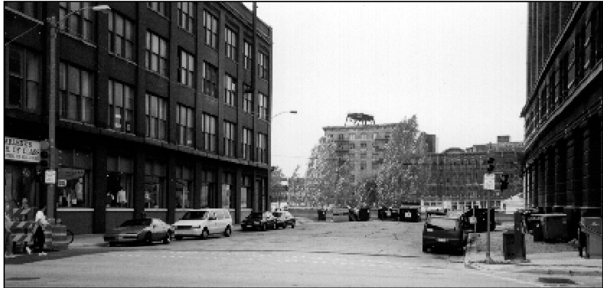
Existing Buffalo St. Stub End Looking West
