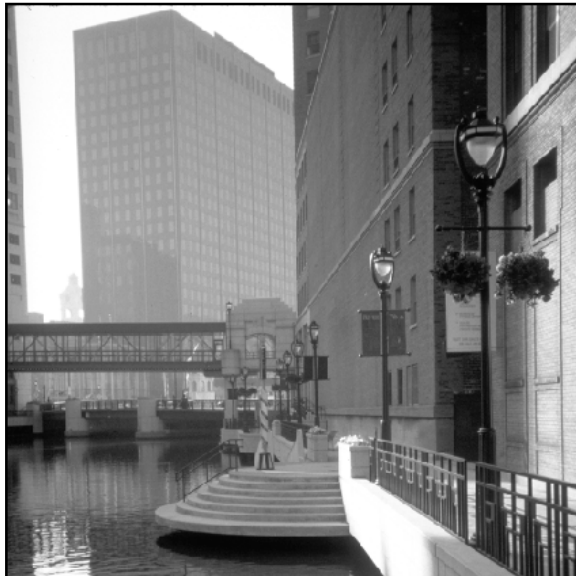
Empire Building Stair on Piles
