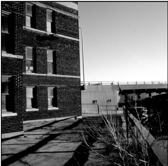
Existing Water St. Bridge Abutment
